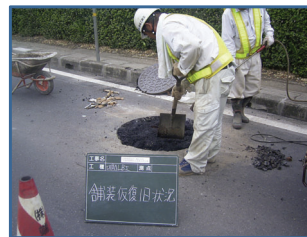
↑復旧材の充填
